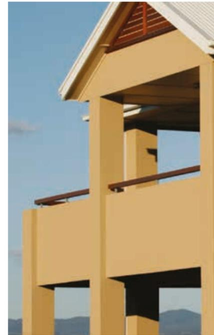
**5** It is important to monitor areas that are heavily exposed to the elements such as parapets and balcony handrail tops. Due to the minimal slope on these areas it will tend to hold dirt and grime which can potentially lead to mould over time if not regularly washed. These building sections should also be checked for any movement over time due to the extremes of thermal movement so it is critical that they are inspected and maintained.
