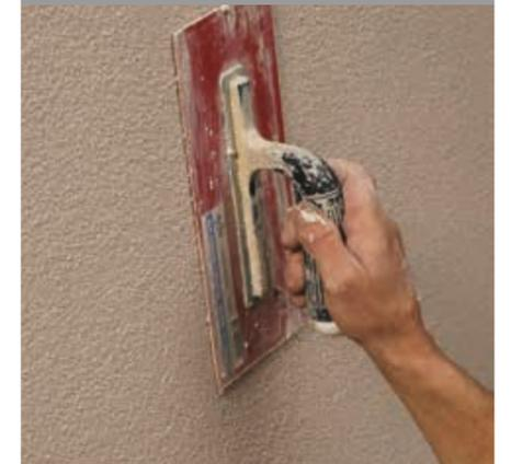
**9** Recoating is recommended after a minimum of 7 to 10 years to rejuvenate the surface appearance. This can be done by using *Dulux AcraTex* elastomeric top coat protective membrane to a selected *Dulux AcraTex* colour which will protect from air pollutants, water ingress and dirt accumulation to provide a new low maintenance surface.
